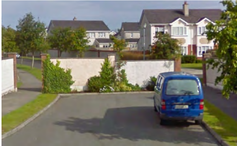
Figure 8.19 Wall to be Removed to Create Bus Gate – Viewed from Kerdiff Avenue
