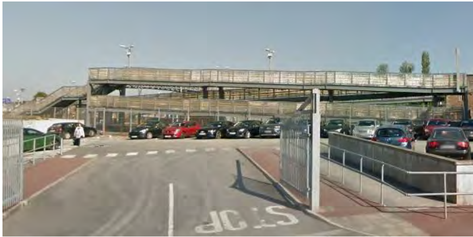
Figure 8.37 Existing Wheelchair Ramp Infrastructure at Sallins Station
