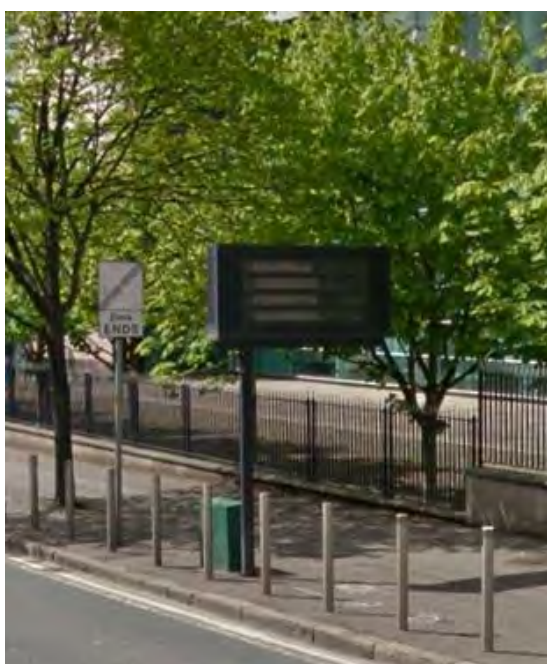
Figure 9.33 Example of Strategic VMS Sign in Oxford Street, Belfast
